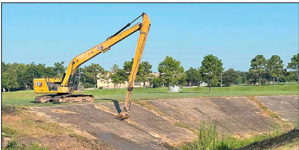
A Fast Action Service Team (FAST) crew from the Harris County Flood Control District was dredging the bayou along near the hike-and-bike trail in Riverstone Ranch this past week. According to county officials, FAST – a dedicated, flexible 29-person maintenance crew – is able to quickly mobilize to handle urgent, localized drainage and infrastructure issues across the county's bayous and channels. FAST duties range from installing signs to completing major channel repairs and erosion fixes.
