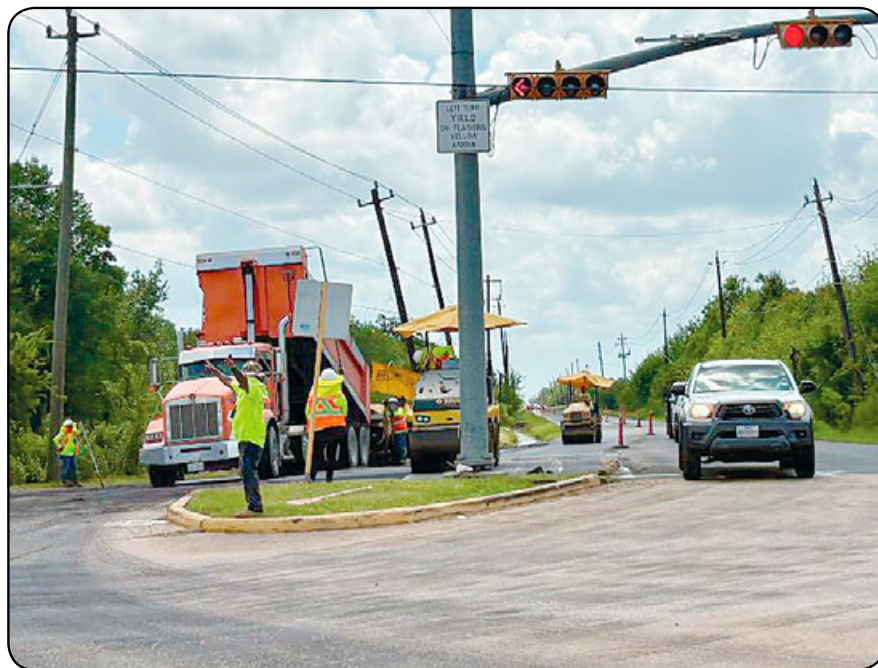
Construction continues along Beamer between FM 1959/Dixie Farm Road and El Dorado Boulevard, where Houston District D City Council Member Carolyn-Evans Shabazz has launched a roadway improvement project. Workers are shown above at Beamer and Dixie Farm. Work is expected to be complete later this month.
