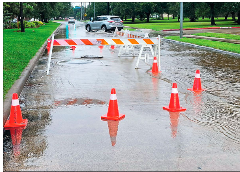
On June 17 and June 20, constables from Jerry Garcia's Pct. 2 office placed traffic cones and barriers around an uncovered manhole to help drivers avoid vehicle damage. Pressure from rain water infiltrating the sewage system caused the cover to be forced off. The manhole is located on Hughes between Sagement Church and Stuchbery Elementary School. See related photo on Page 1.
