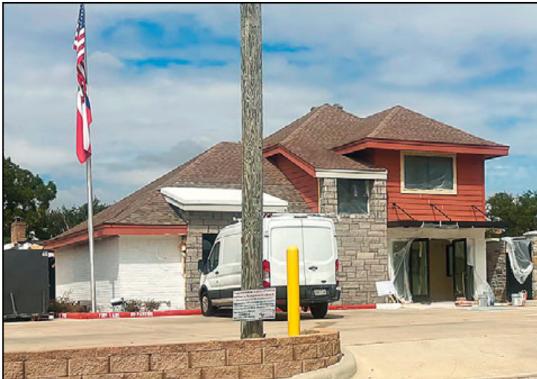
Construction recently resumed on the Sagemeadow MUD building, located on Hall Road at Blackhawk, after being dormant for several weeks. MUD officials said the work is needed to upgrade the 50-year-old building's aging infrastructure, as well as to provide additional security for staff members.
